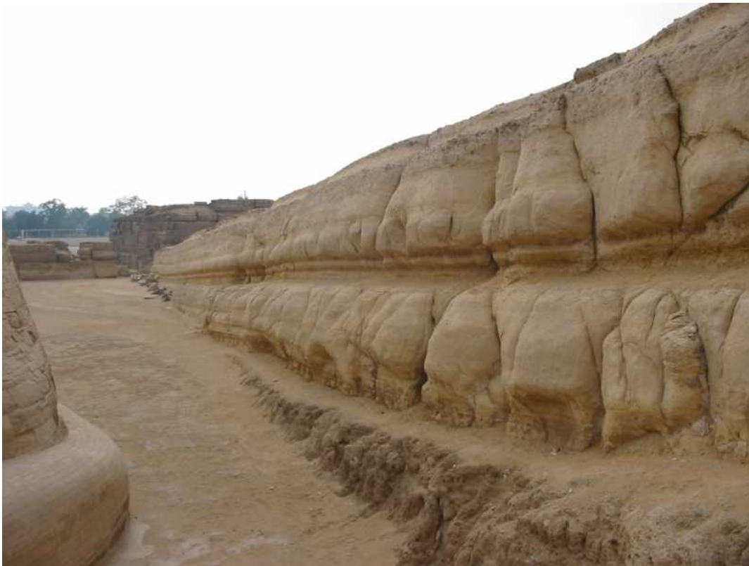
Figure 92. Rain erosion of the walls of the Sphinx enclosure
